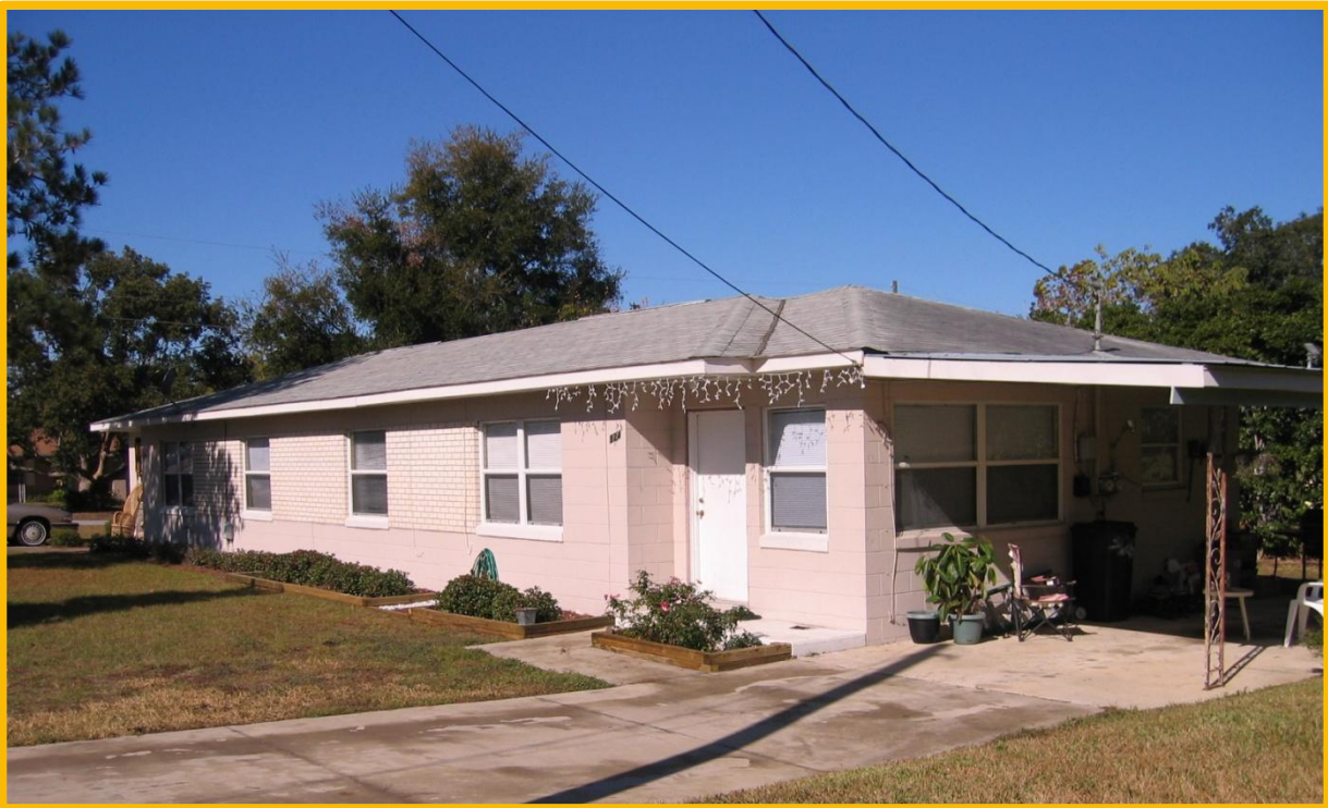
View looking Northwesterly
