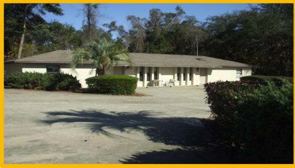
Exterior View Typical Unit Duplex
